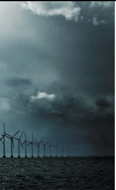
At Middelgrunden off the coast of the Danish capital, Copenhagen, 20 wind turbines are installed in a slight curve with 180 meters distance and a total length of 3.4 kilometers. The total area is about 1 hectare. The 20 x 2 MW wind turbines at the off-shore wind park are equipped with 3 x BSFH 330 Monospring brakes with Sintermetal brake pads supplied by Svendborg Brakes. The 2MW turbine is a stall-regulated machine with a rotor diameter of 76 meters.
