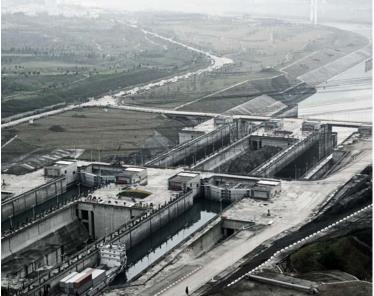
The dam's ship lift will shorten the time taken for ships to pass the dam from three hours to one. Svendborg Brakes became the chosen provider of among others 32 brakes acting as parking brakes, respectively security brakes for the electrical drive.
