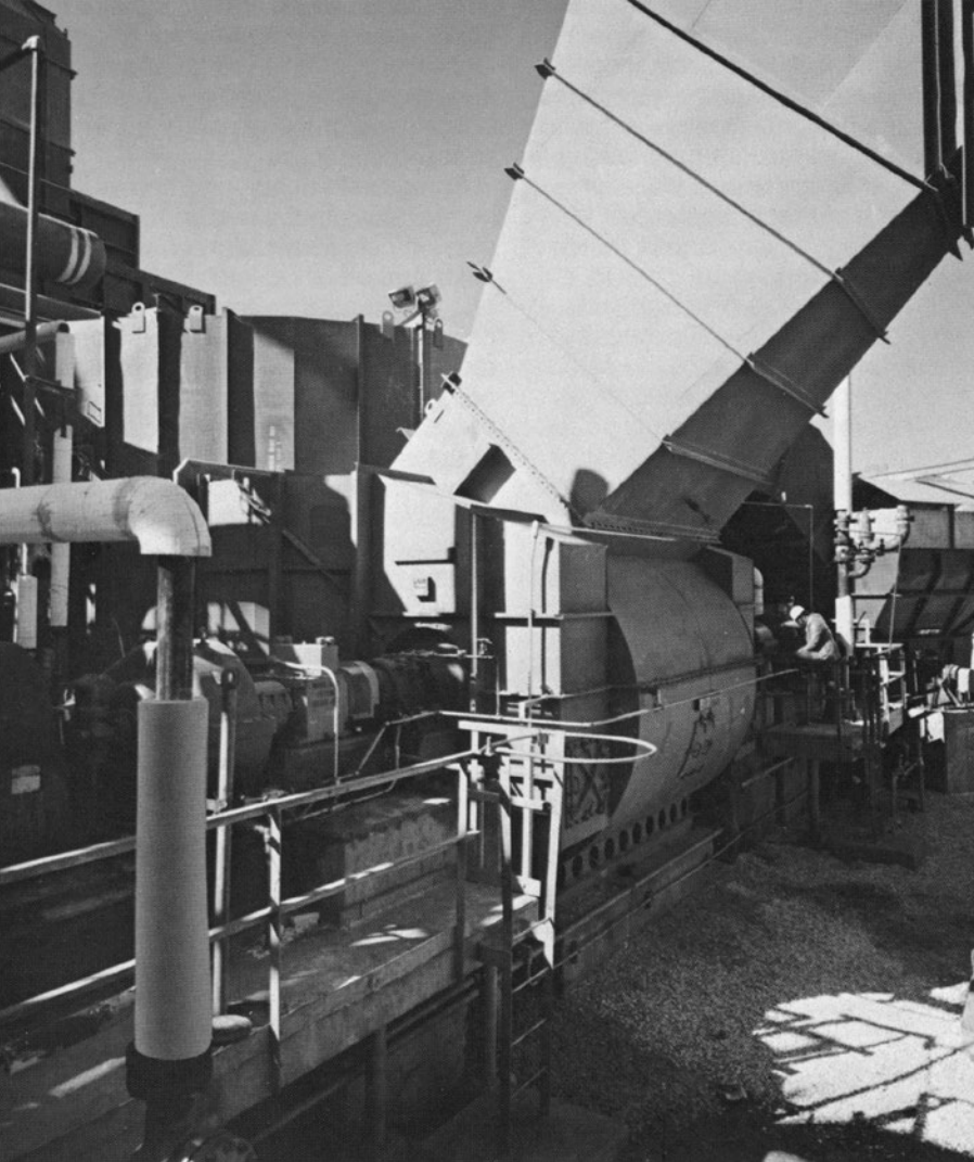
Photo: Dual driven induced draft fan through Marland CECONS to provide process steam at a Southern chemical plant
